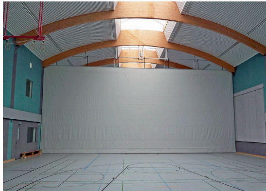
Partitioning curtain mounted on laminated wood truss
