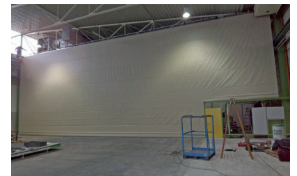
Industrial buildings can also be partitioned. Cutouts and simple wicket doors at the end of a curtain are possible and often necessary to secure the escape routes in case of fire.
