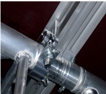
Platform fastening to trusses
