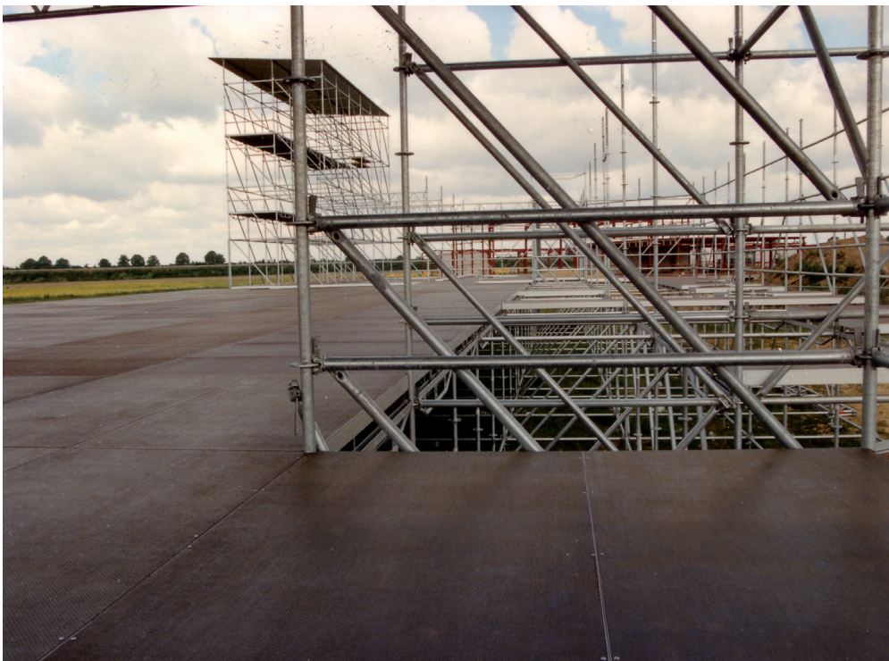
Example: Scaffolding with BÜTEC platforms as stage floor and integrated roof.
