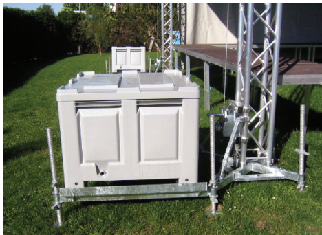
Ballasting with water tanks and booms
