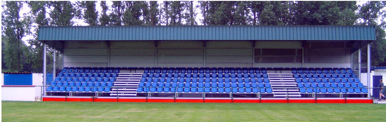
Stand roofing and stadium grandstand composed of plug-in leg platforms with screen print plate and PVC bucket seats
