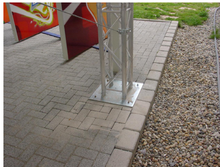
Anchoring to the ground with impact dowels
