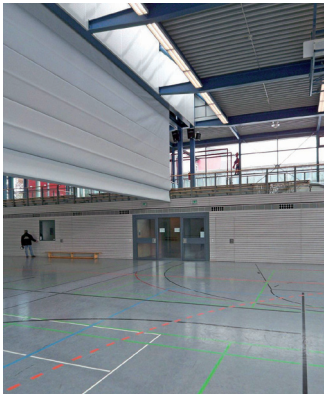
on double steel truss
