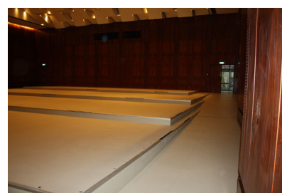
completed platform area
