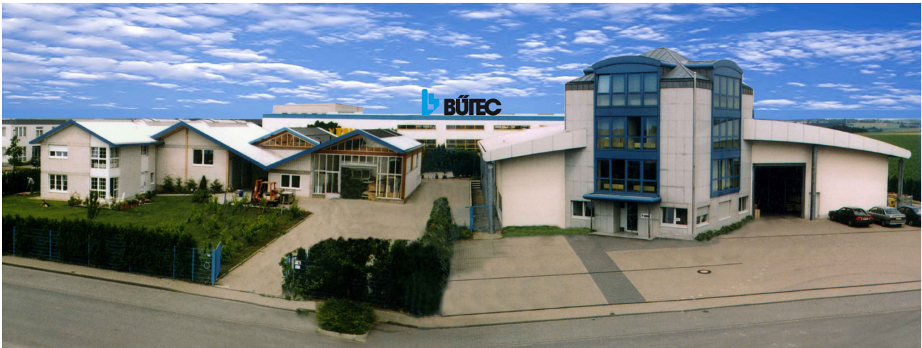
BÜTEC operational and administrative buildings with four production halls in Mettmann.
