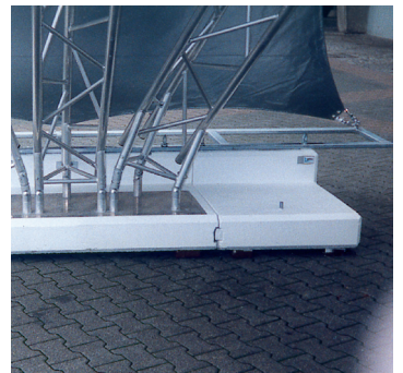
Ballasting by installation on pre-cast concrete
