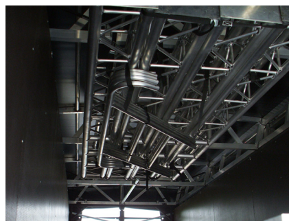
For transport, struts and railings are attached to the roof supports.
