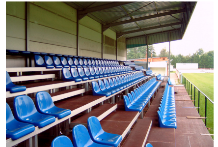
PVC seat shells on stadium grandstand
